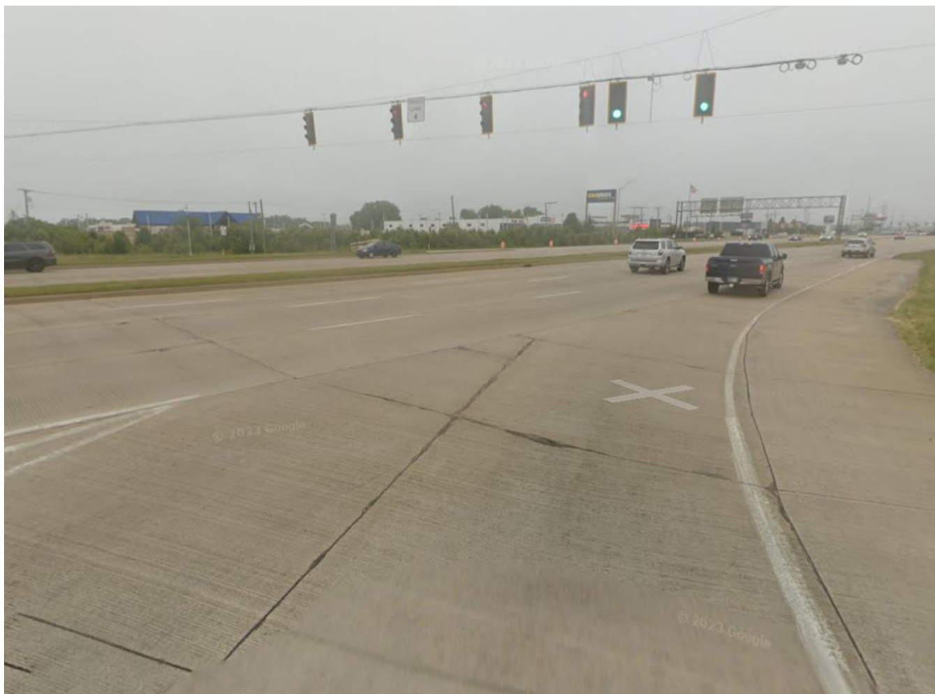
Figure 31: Ambiguous Pavement Markings at an Offset Intersection
